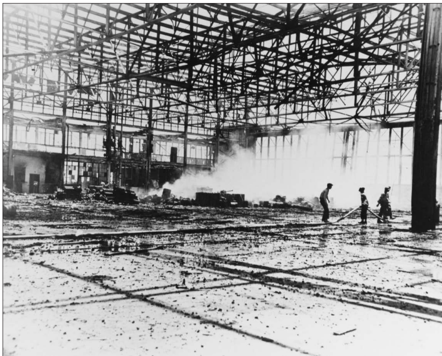
Interior of one of the Midway hangars after the Japanese raid.
